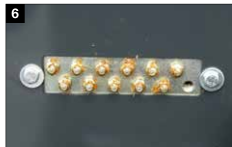
Centralized grease banks for roller bearings
