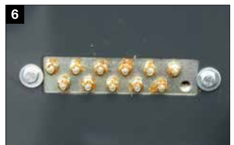
Centralized grease banks for roller bearings
